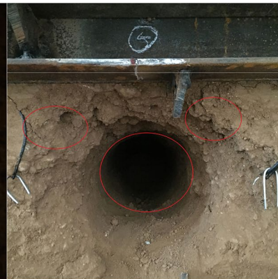
(c) Shear failure with an X-shape and particles falling from the roof
