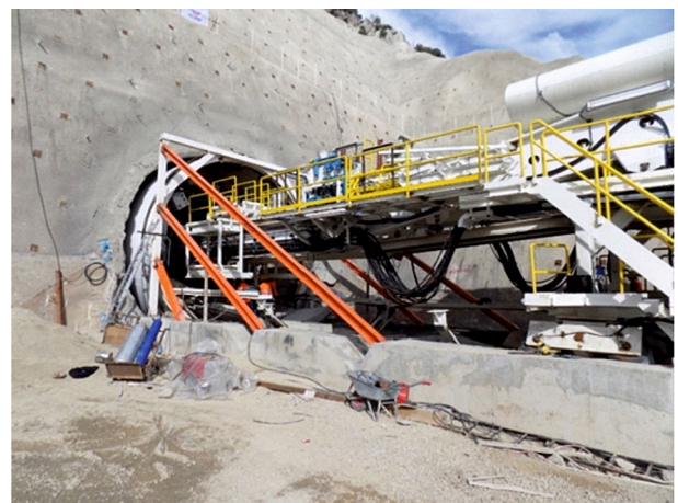
Fig. 6 The conveyor belt system of the TBM
