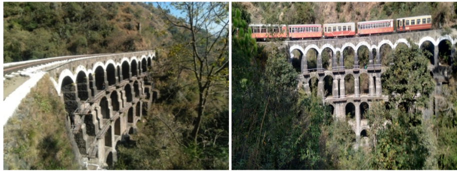
(a) Photograph of Bridge No. 541, Kalka Shimla Mountain Railways
