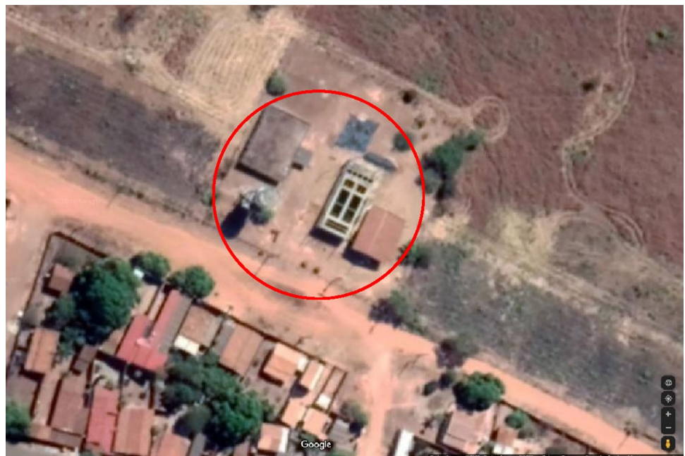
Fig. 2 General view of the location of the water treatment plant and treatment units
