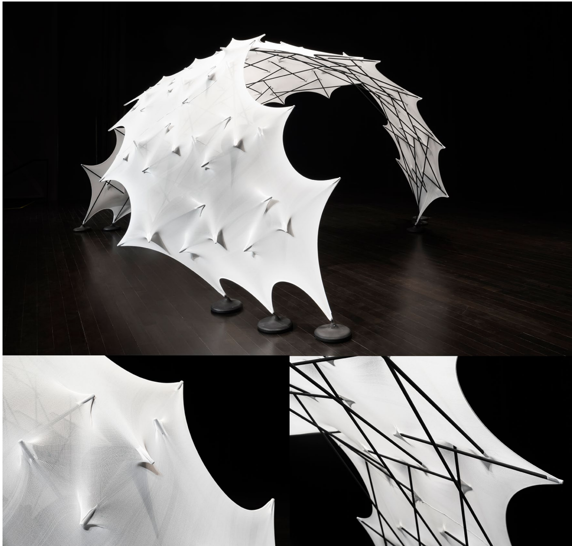
Fig. 13 Knit tensigrity shell at the IASS Form&Force Expo 2019. Photo Credit: Katariina Träskelin
