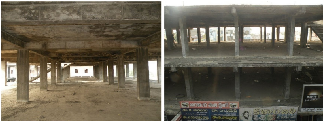
Fig. 2 Photographs of the existing RC frame building
