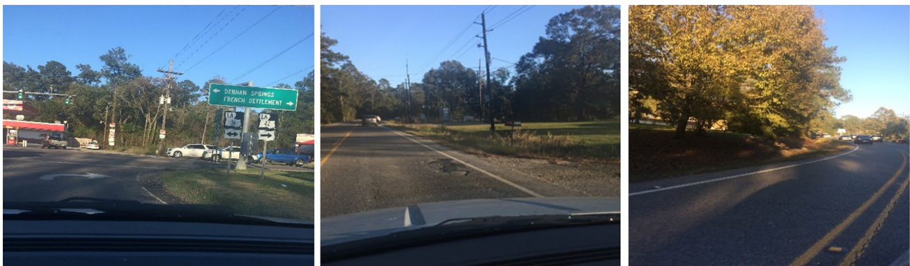
Fig. 5 Existing road conditions of LA 16 and LA 42
