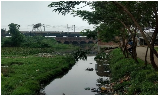
Poor drainage system
