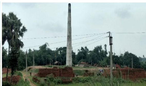
Brick kiln factory in agricultural field
