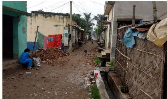
Mud road with improper drainage
