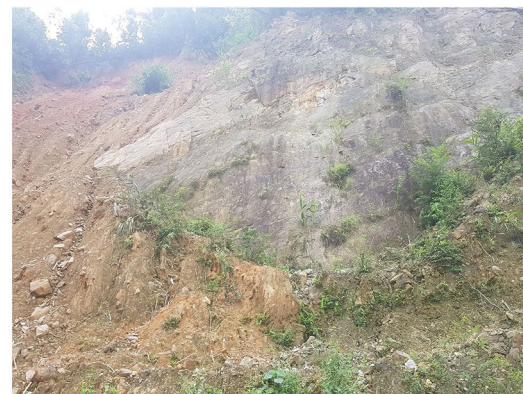
Very high level of landscape erosion
