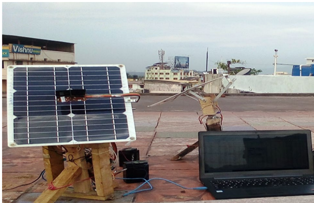
Fig. 6 Dual axis solar tracking system and fixed panel
