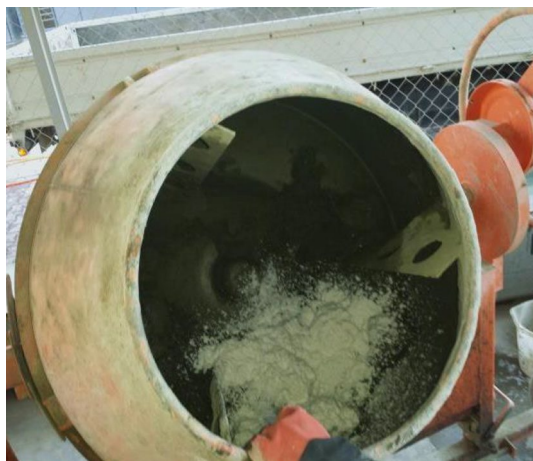
Plate 3 Addition of foam to the mix
