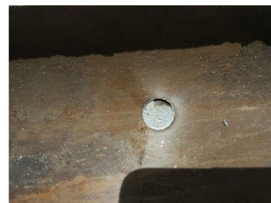
Fig. 13 Real topography of the artificial hole
