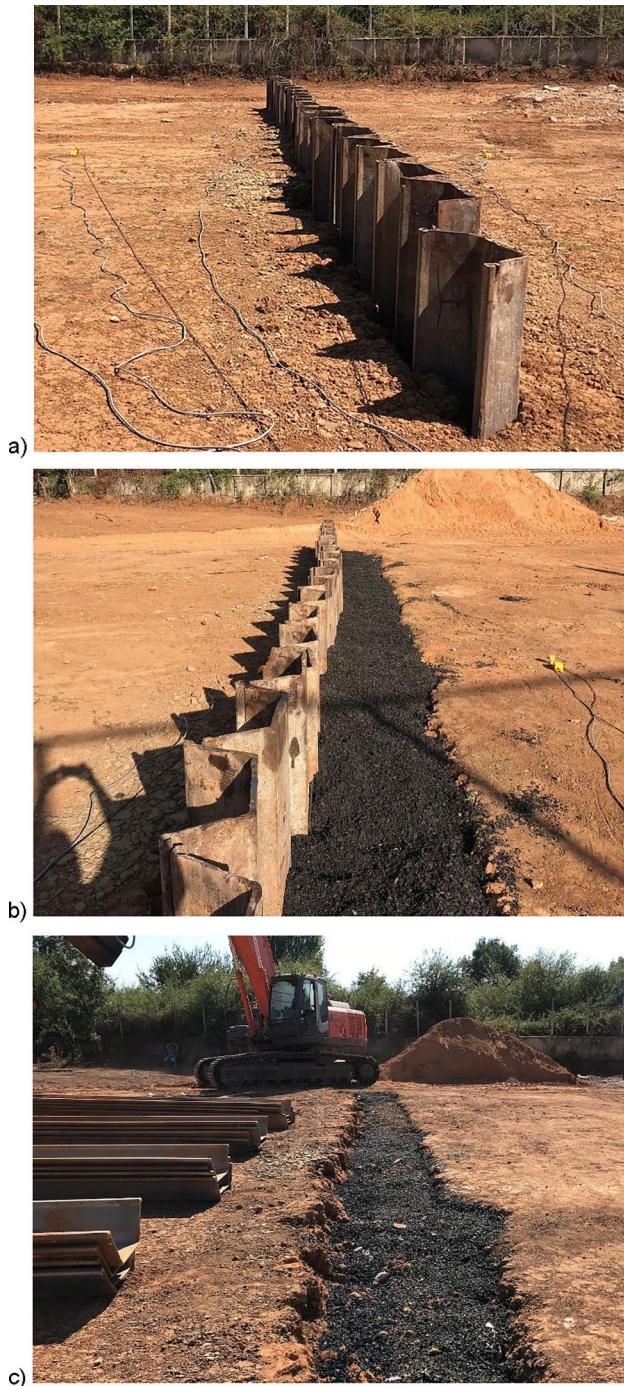
Fig. 4 Wave barriers a sheetpile b rubber chips-sheetpile coupled barrier c rubber chips
