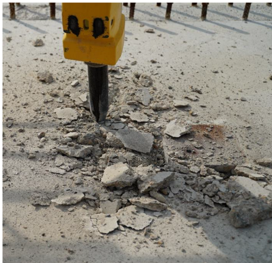
(a) Snapshot of the deconstructed area.
