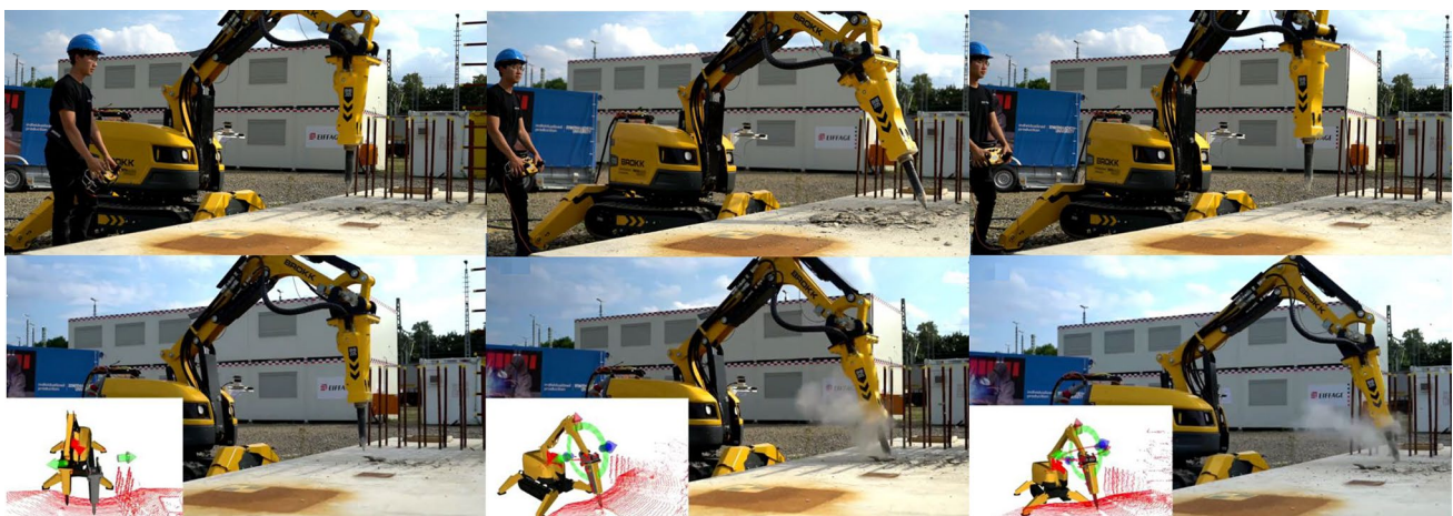
Fig. 13 Snapshots of the manual teleoperation (top) and the semi-autonomous approach (bottom) for deconstruction
