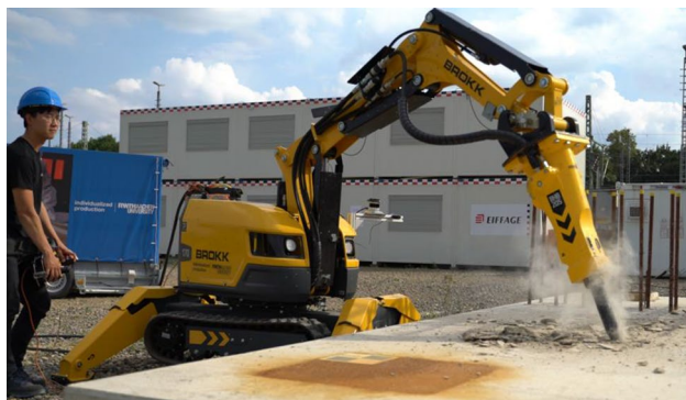
Fig. 1 Conventional teleoperation, where the human operator directly stands on the deconstruction scene
