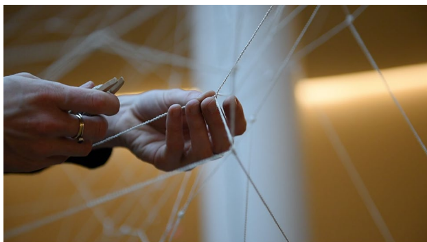
Fig. 8 Super Munter Hitch knot. The Super Munter Hitch knot was used to create connections that were steadfast—especially in combination with the textured filament surface—and easily undone. Hitches made during the first layers featured two full turns, whereas those made during the densification process featured only one
