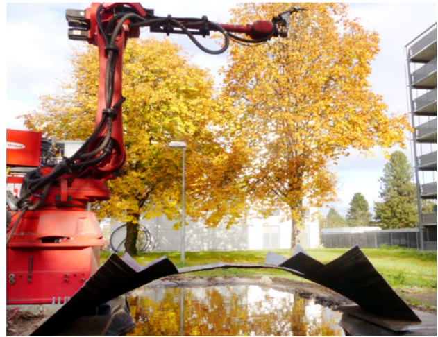
Fig. 17 Picture from construction site
