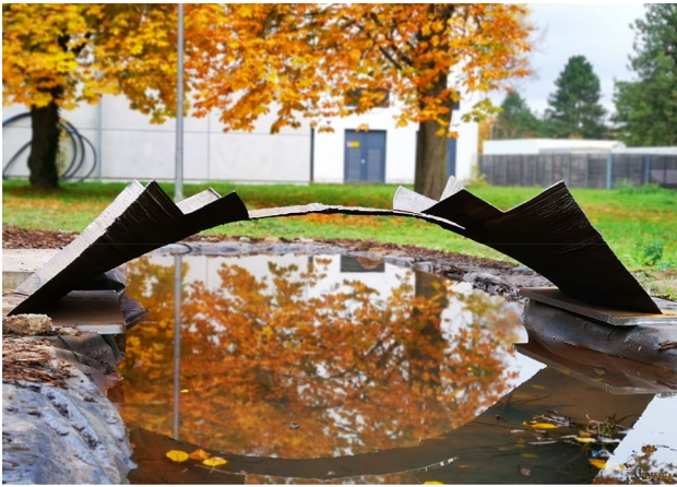
Fig. 23 Bridge shortly before being disassembled
