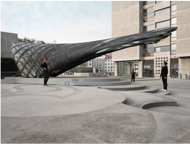
Fig. 15 Final 12 m long composite cantilever
