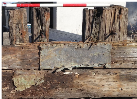
Fig. 16 Detail of intact section showing double framing, two hull planks, and preserved Muntz-metal sheets at GCCC depot (remains are photographed upside down; the caprail is attached to the bottom of this assembly and not visible in photo). (Photo by Lauren Davison, 2014.)
