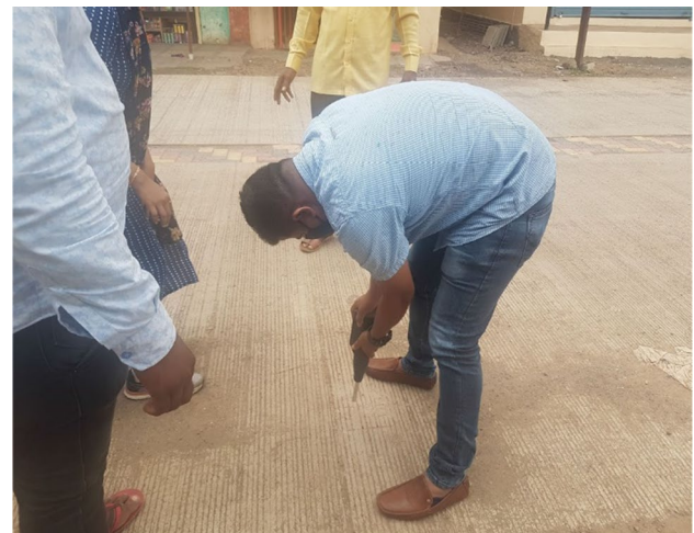
Fig. 7 Rebound hammer test
