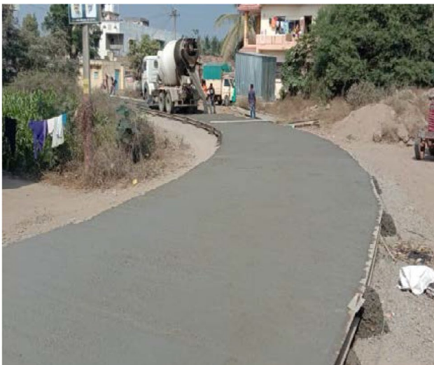
Fig. 3 Laying of PQC
