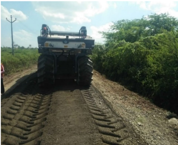
Fig. 2 Recycling of base course with Recycler
