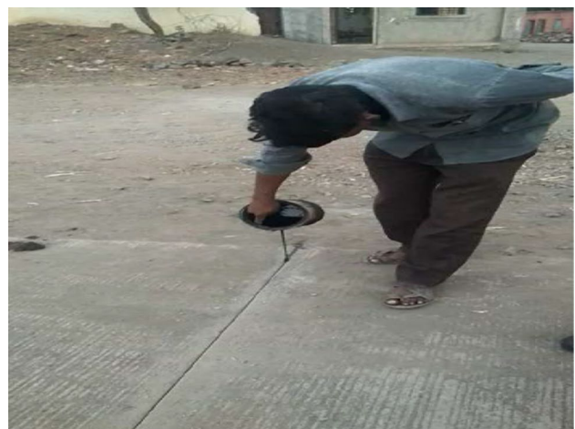
Fig. 5 Joint cutting and filling with sealant
