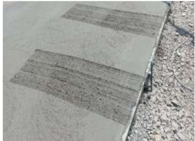
Fig. 4 Texturing of concrete
