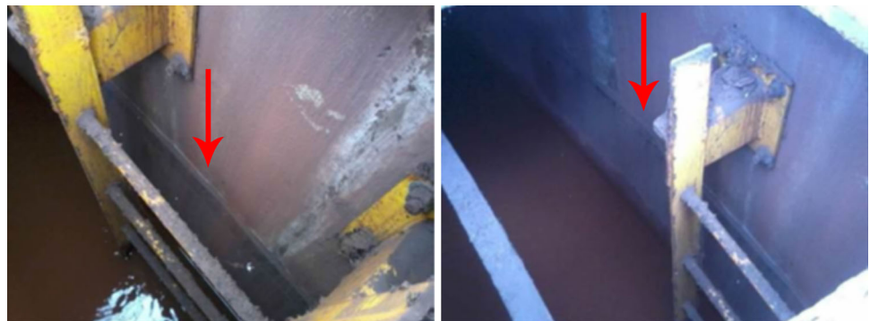
Fig. 8 Limit of the internal waterproofing approximately 60 cm below the top of the structure. We also observe the color of the water
