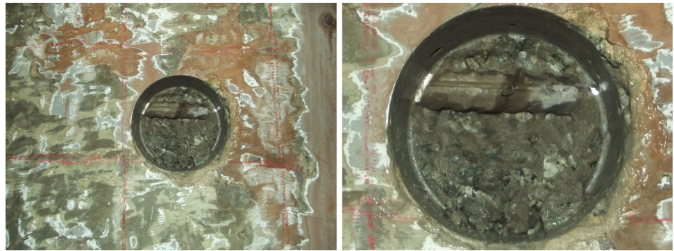
Fig. 6 Detail of rebar built into the concrete
