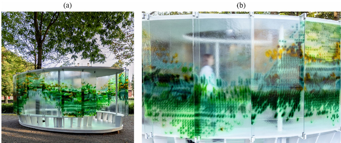
Fig. 1 Views of the pavilion with polychromatic kilned glass panels showing (a) the relationship to the surroundings through the decorative pattern applied and (b) the graded transparency obtained through the colour grading process. Images credit: Digital Building Technologies, ETH Zurich; Photographer: Evangelos Roditis
