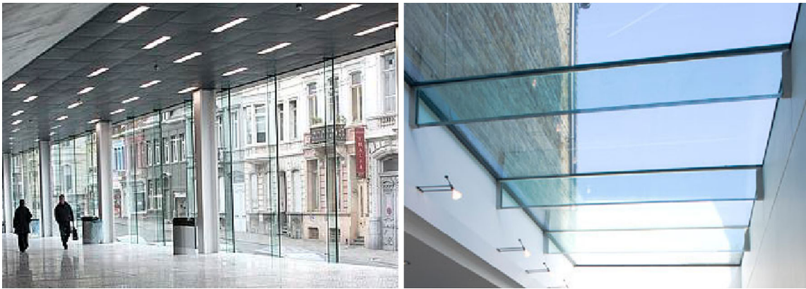
Fig. 1 Examples of beam-like element in facades ( left ) and roofs ( right ). The photos are reproduced from Christiaens (2009) and Giles Pike Architects (2016)
