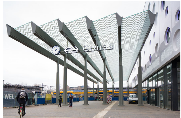
Fig. 8 Gouda train station canopy
