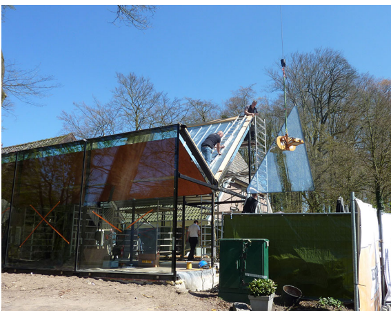
Fig. 1 Situation during construction of De Boerderij
