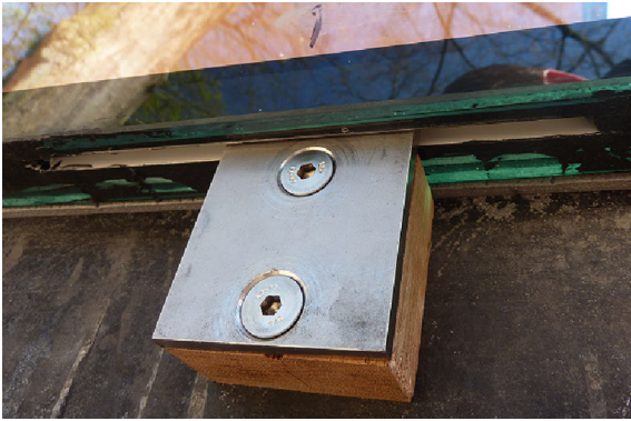
Fig. 6 Horizontal fixation of the glass
