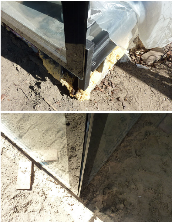
Fig. 7 Corner detail: during construction ( top ) and after closing ( bottom )
