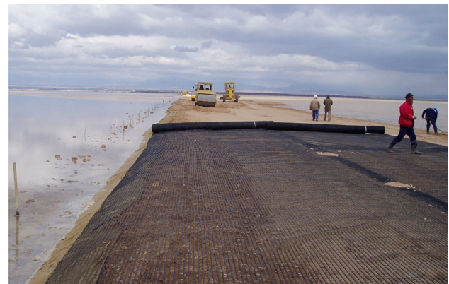
Fig. 7 Laying the biaxial geogrid over the first lift of embankment
