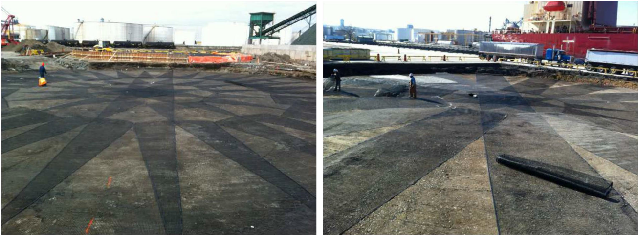
Fig. 11 Geogrid reinforcement on excavation base
