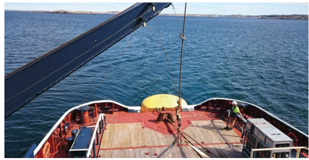
Fig. 4 Simultaneous installation of L12D with its buoy [36]
