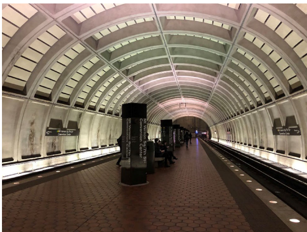
Figure 1 “High-dome” structure widely used in stations of the metro system of Washington, D.C.
