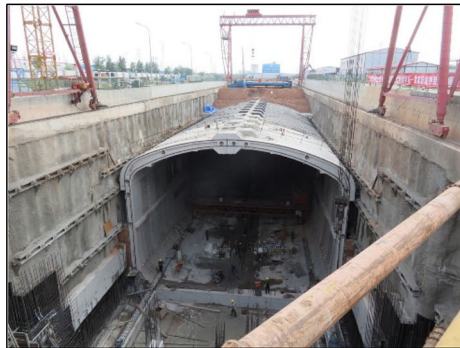
(c) Completion of structure
