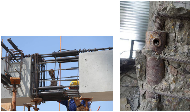
Fig. 6 Rebar splicing by grout-filled coupling sleeve and typical deviation
