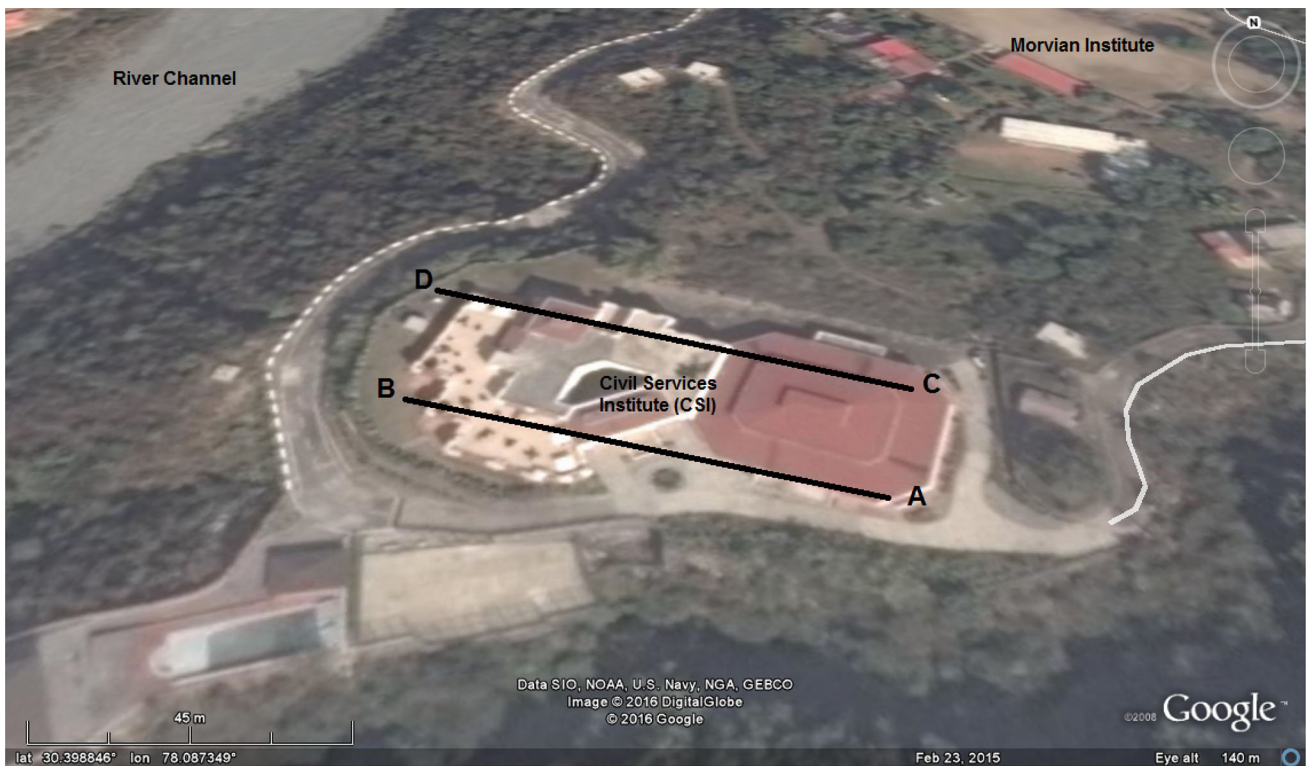
Fig. 2 Field Location Map of the study area with ERT profiles on Google map
