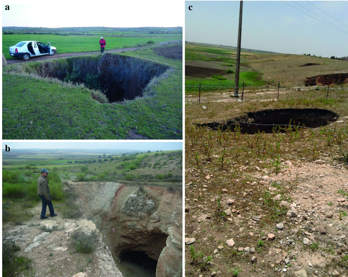
Fig. 1 Some of collapse dolines in the study area. a This collapse doline occurred in 1996 at the bottom of Oulad Sidi Allal Ben Jeddi polje. b This collapse doline shows the gypsum beds of Upper Jurassic, in the background of the photo you can see the precedent
