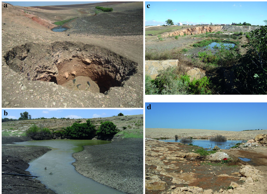
Fig. 8 Aggravating factors observed in the study area (a) a collapse doline detected near a swallow hole where the wastewaters of Jemaat Shaim city are discharged (b) the drainage of surplus irrigation water by injecting directly into a collapse doline near of the Moul El Bergui
