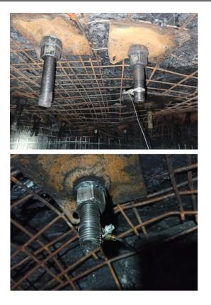
Fig.9 The investigated rock bolts in an underground opening in a working coal mine
