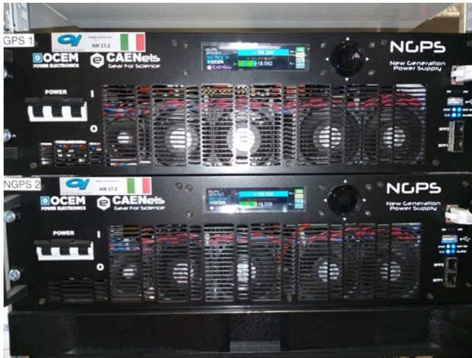
Fig. 18 Quadrupole power converters
