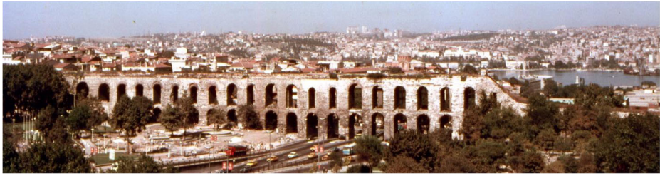
Fig. 4 Valens (Bozdoğan) aqueduct in the East Roman / Byzantine capital Constantinople (İstanbul) (photo:Ü.Öziş)
