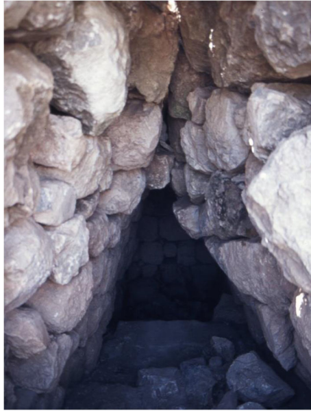
Fig. 2 Springwater collection chamber in Hattusha (photo:Ü.Öziş)
