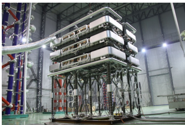
Fig. 12 1,000 MW/ \pm 320 kV HVDC Flexible converter valve
