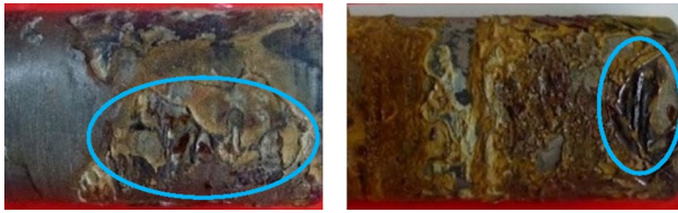
Fig. 1 Different degrees of corrosion on an MP near an electrified railway
