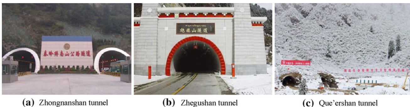
Fig. 2 Typical highway tunnels in China
