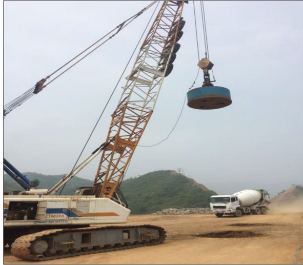
Fig. 7 Dynamic compaction machine in the project
