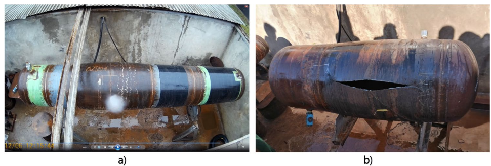
Fig. 18 The burst test of the DN600 pipeline sections: a end of the burst test (recorded from above) of the FSPS7 pipeline section; b the FSPS8 pipeline section after the test
