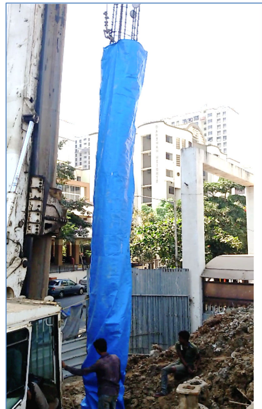
Fig. 8 Geofabric pile liner with LDPE melt coating
