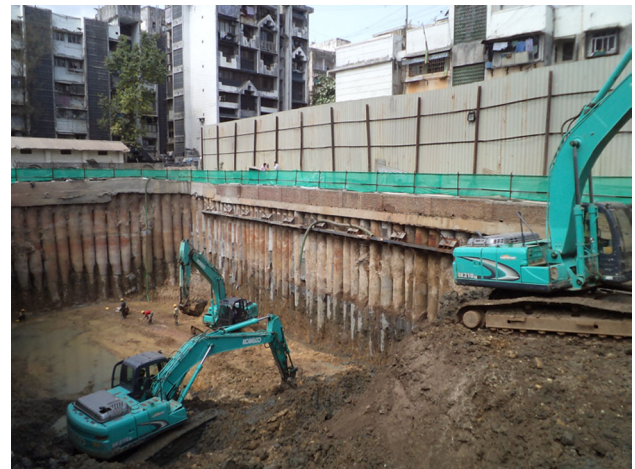
Fig. 19 Properly designed shoring piles with anchors
