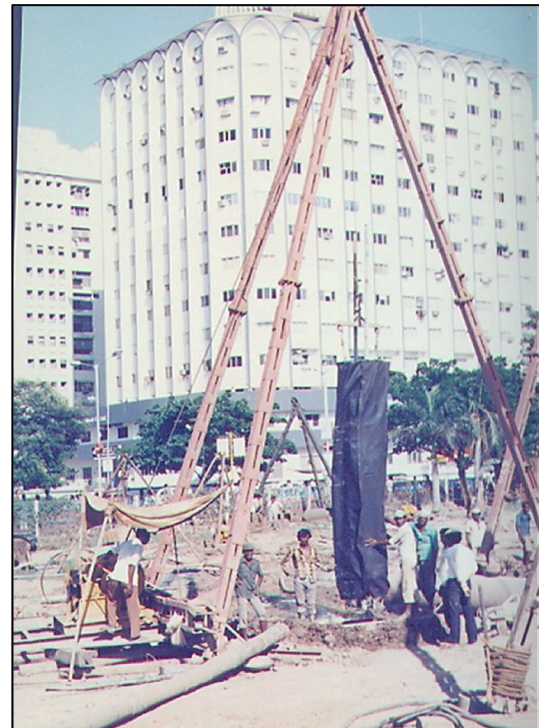
Fig. 7 Geofabric pile liner with bituminous slip coating
