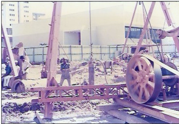
Fig. 10 Airlift cleaning of pile tip
