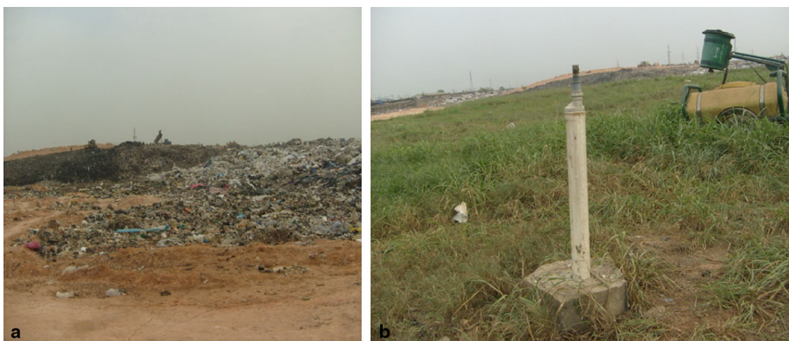
Fig. 4 Portions of the Olusosun landfill (a partially capped areas; b a well-head for LFG capture)
