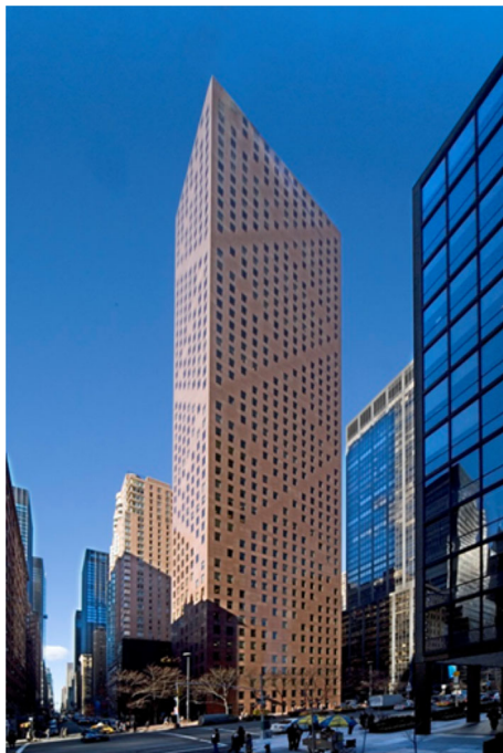
Fig. 5 Braced tube system; 780 Third Avenue building
