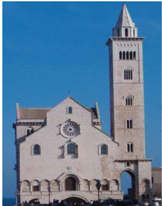
Fig. 1 Trani's Cathedral and its bell tower
