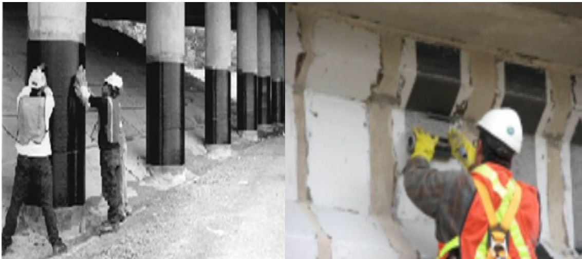
Fig. 2 Practicing strengthening of RC girder by CFRP laminate (Alferjani et al. 2014)
