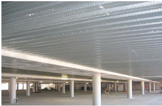
(a) Soffit of a one-way composite slab and beam floor system
