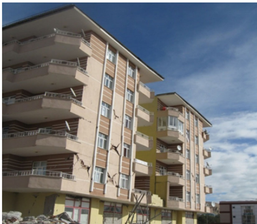
Fig. 1 A view of the prototype building
