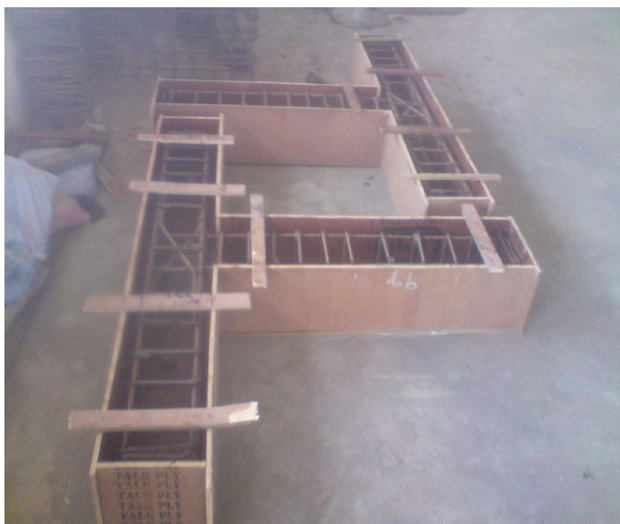
Fig. 3 Formwork and reinforcement
