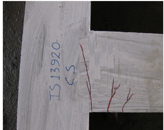
Fig. 11 Crack pattern of IS 13920 CS
