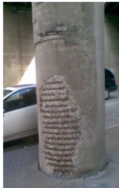
Fig. 2 Bridge column, Howe Ave., Akron, OH, USA
