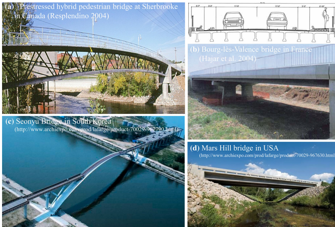
Fig. 17 Examples of UHPFRC applications in bridges.
