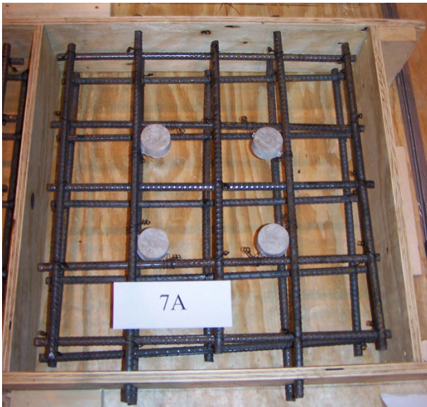
Fig. 5 Placement of embedded galvanic anodes.
