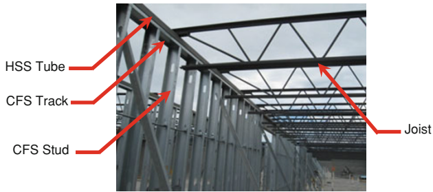
Fig. 1 Light-gauge steel framing.
